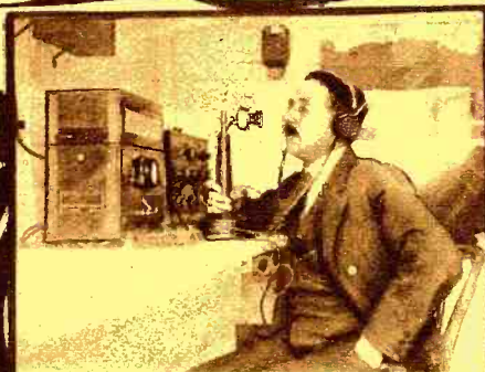
Above (Left) P. D. Powell, of the Bureau of Standards, Has Evolved a Radio-Receiving Set in Which the Usual Batteries Are Eliminated and Necessary Current Obtained from Electric Light Line. It Is Claimed There Is No Hum.
